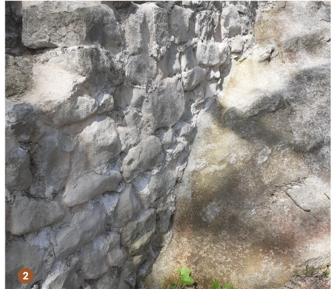
(frontal view of a part of the wall)
